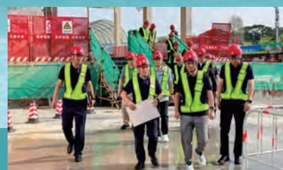
視察設安全防控措施落實情況 Inspecting the implementation of safety control measures
