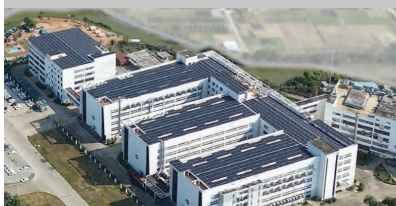
Town Ray's installation of a solar photovoltaic system at its Huizhou production facility is a key initiative supporting the company's goal to reduce Scope 2 emissions and transition toward renewable energy sources. 登輝在惠州生產基地安裝的太陽能光伏系統，是推動實現範圍之碳減排及向可再生能源轉型目標的重要舉措。
